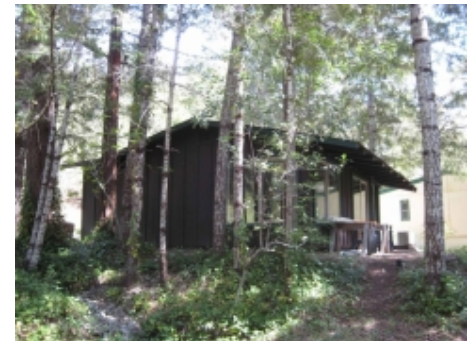
The newly remodeled Tara Cottage.
